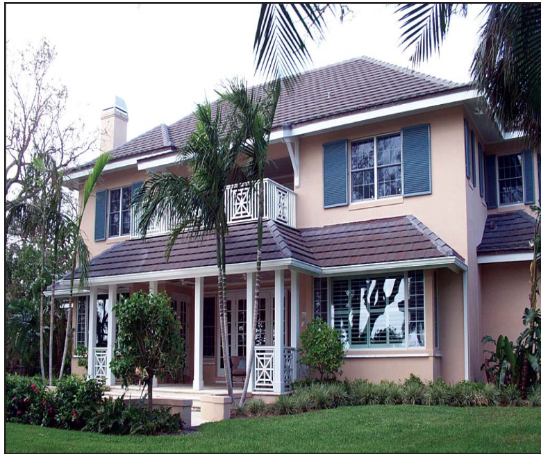
The original house became the second story when this elevation project was completed. The finished home is one foot above the Base Flood Elevation and has storm shutters for all windows.
